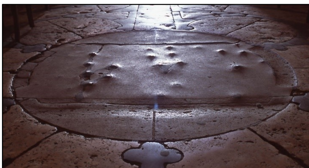
Central panel of the Chartres labyrinth, showing the rivets that held the former plaque in place. Photo: Jeff Saward/Labyrinthos
