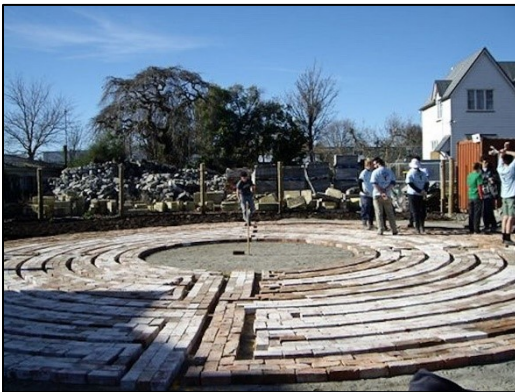
The labyrinth under construction Photos: Jenny Drury, 2012
